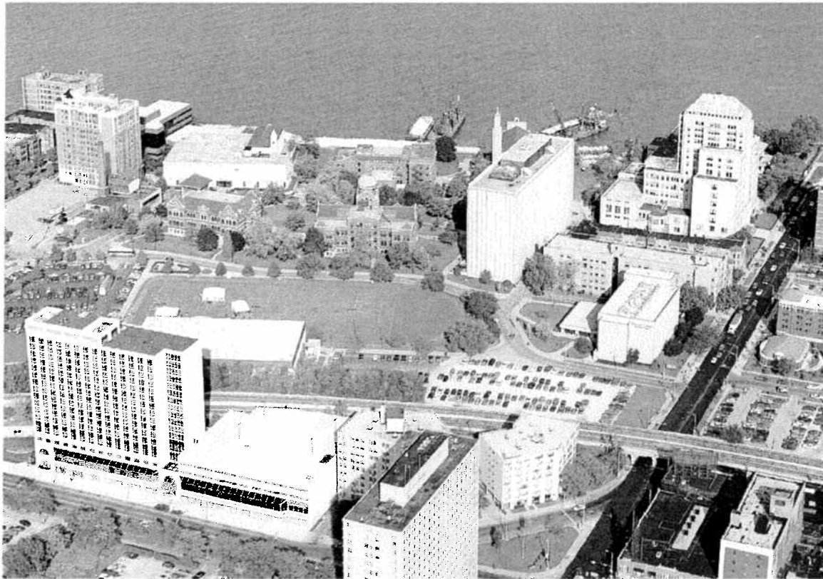
The Mundelein College Skyscraper Building is significant as an important building for Roman Catholic higher education in Chicago for more than 70 years, first as the headquarters for Mundelein College, then as an important building owned by Loyola University Chicago. Top right: Mundelein students going to classes in the 1950s. Top right and bottom: The building, now known as the Mundelein Center, as it appears today.
